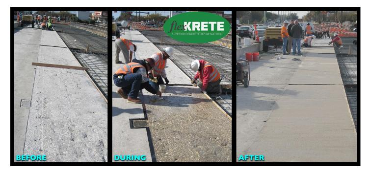
The above image illustrates how an existing sidewalk became part of a bridge expansion project. Using FlexKRETE as an overlay material strengthens the surface, making it suitable for vehicular traffic.
